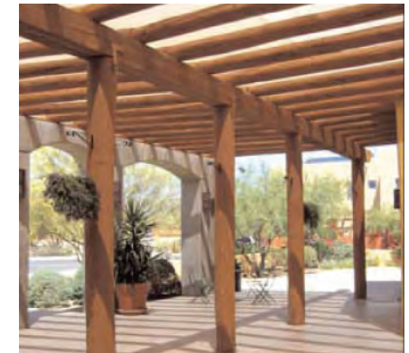
Rough-sawn wood details
