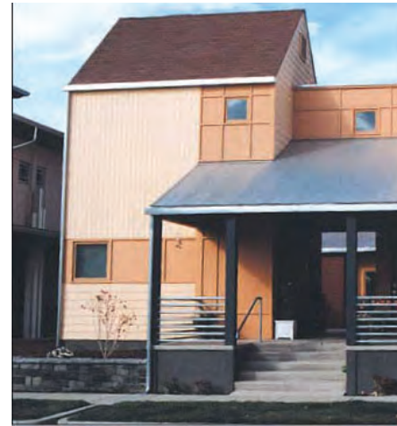
Composition of different wall cladding
